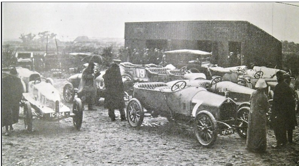
Car enclosure, 25hp Talbot on left
